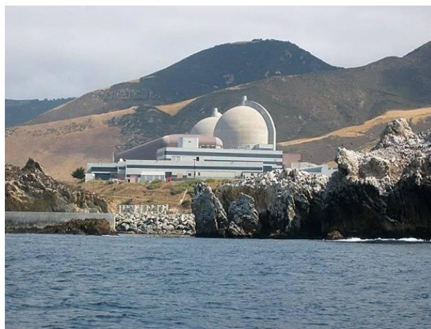
Diablo Canyon Nuclear Power Plant, San Luis Obispo, California
