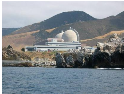
Diablo Canyon Nuclear Power Plant
